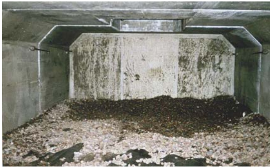
Minocqua, WI, MCTT filtration/sorption chamber
