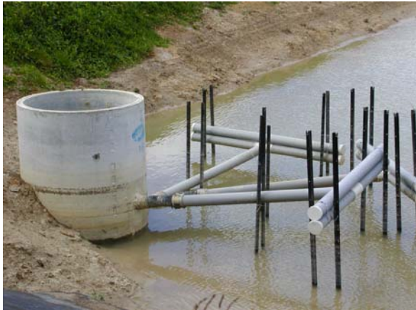
Floating, multi-stage risers at Auckland, NZ, construction site pond
