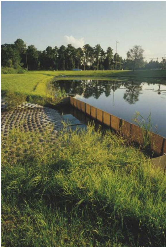
Orlando, FL, pond modifications to capture litter and other floating debris in pond
