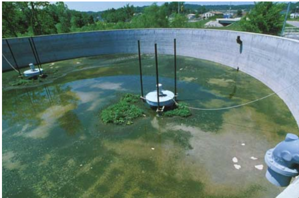
Moody, AL, storage tank for capture of SSOs prior to treatment plant
