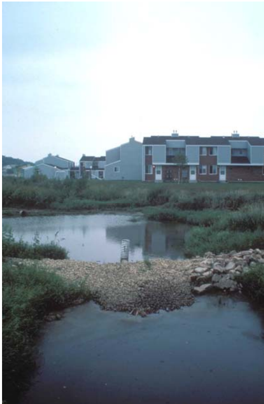
Gravel emergency spillway over riser and culvert, Madison, WI
