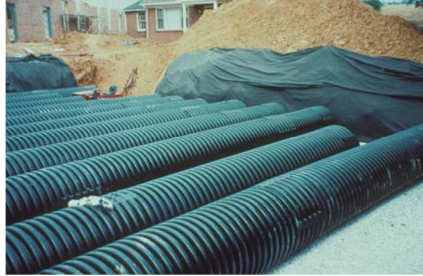
Underground plastic pipe detention facility during construction
