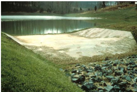
Large concrete emergency spillway
