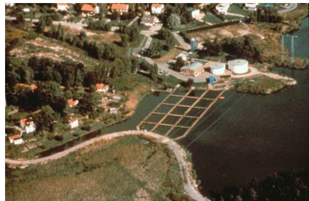
FBM installation in Sweden (Karl Dunkers photo)
