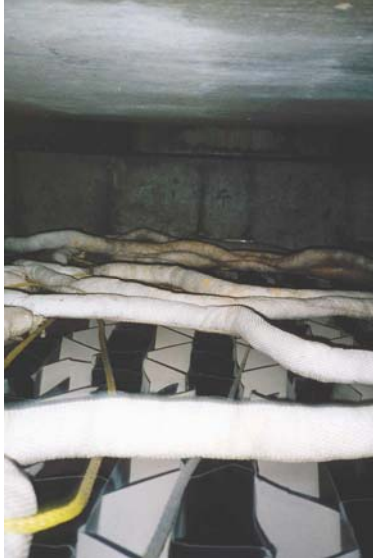
Ruby Garage, Milwaukee, WI, MCTT main settling chamber
