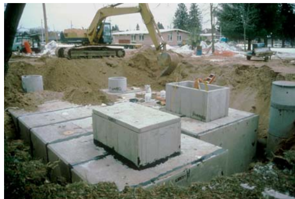
Construction of Minocqua, WI, MCTT
