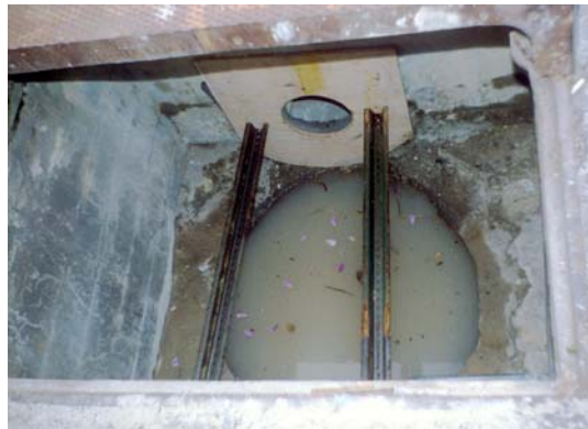
Retrofitted sump at inlet to provide capture of sediment as catchbasin
