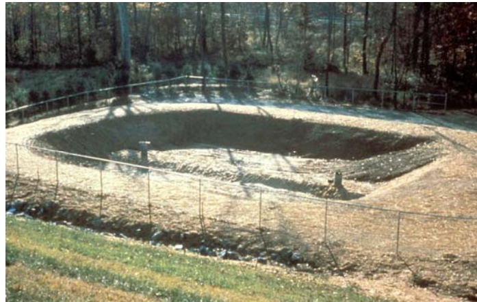
Typical dry pond with fence and steep slopes
