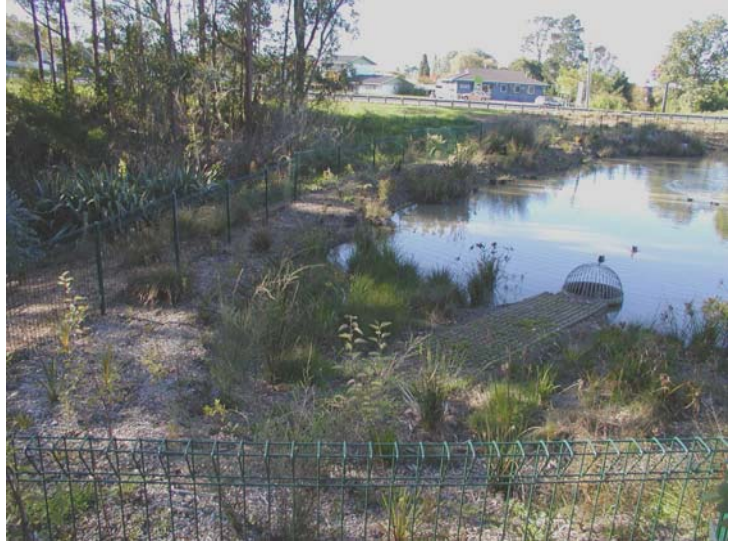
Auckland, NZ, pond in cemetery serving surrounding residential area
