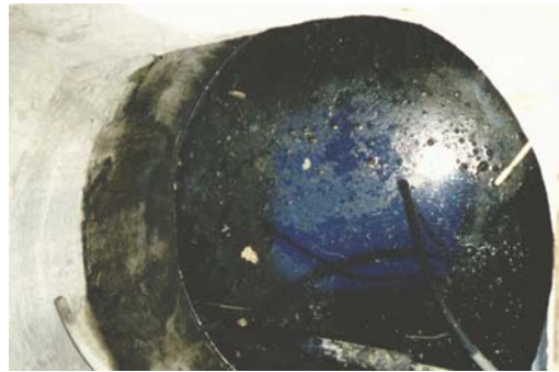
Ruby Garage, Milwaukee, WI, MCTT inlet chamber
