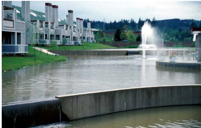
Lake Oswego, OR, pond treating runoff from adjacent shopping center and apartment complex
