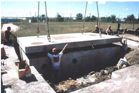
Construction of Ruby Garage MCTT
