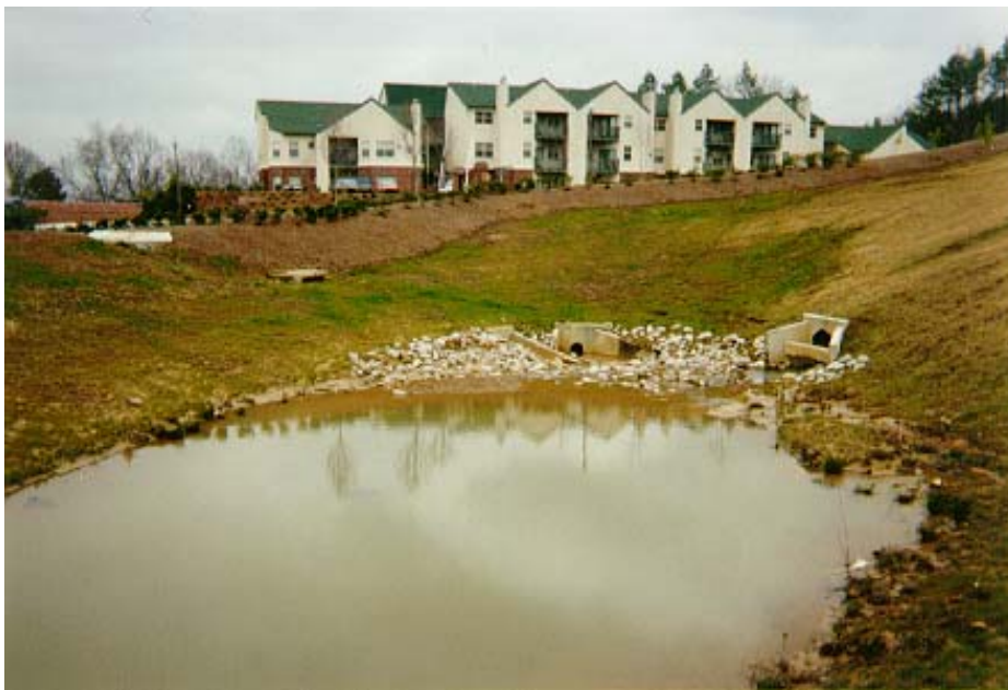
Figure 125. Facing north, from left to right: emergency spillway, secondary outlet, primary outlet, large inlet.
