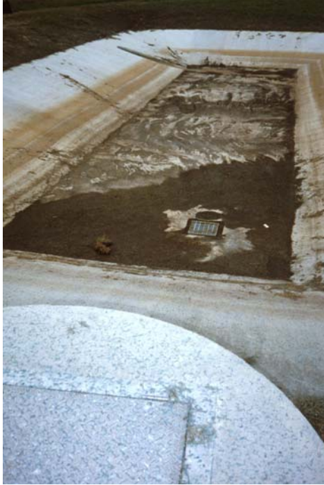
Austin, TX, dry pond prior to horizontal flow sand filter
