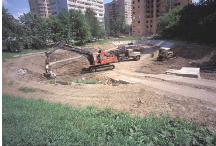
Rebuilding pond and removing old sediment at apartment housing, Moscow, Russia
