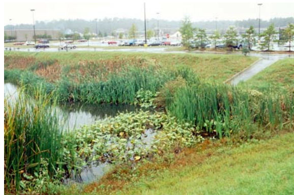
Birmingham, AL, shopping center pond, showing vegetated safety ledge
