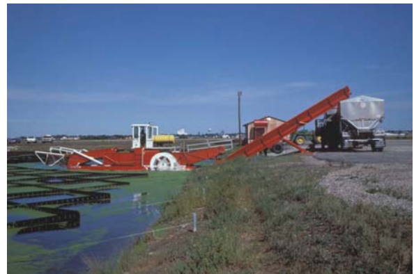
Engineered vegetation removal system at stabilization pond (Lemna Corp. photo)
