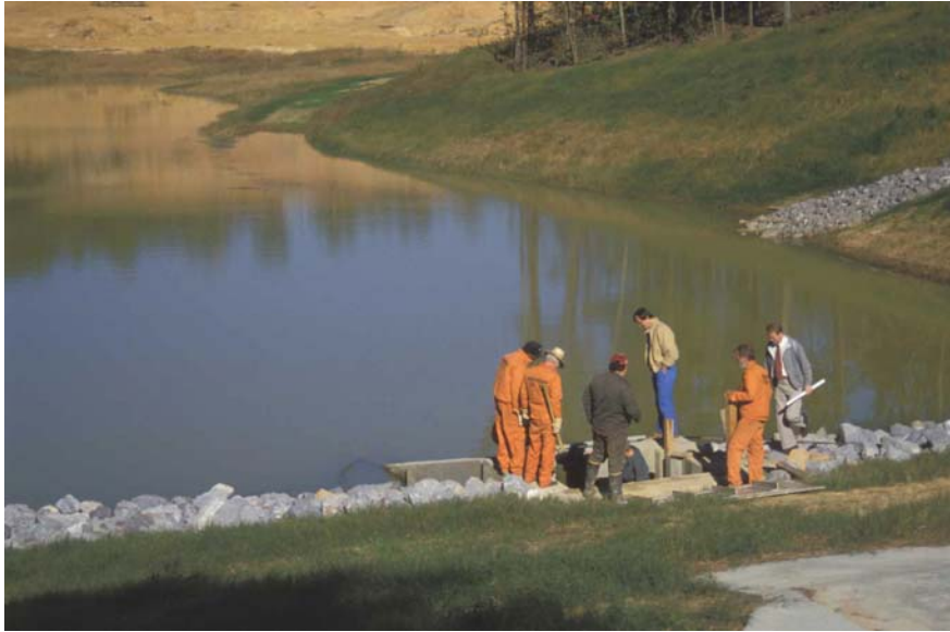
Figure 29. Maintenance inspections and cleanout at outlet of a Birmingham, AL, pond.
