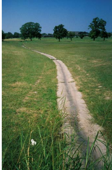
Madison, WI, golf course dry pond with concrete pilot channel
