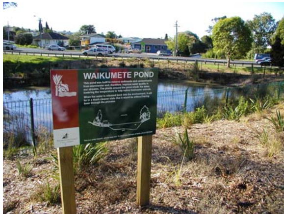
Auckland, NZ, sign explaining function of wet pond treatment
