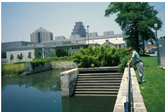
Downtown Austin pond, following oil and grease trap
