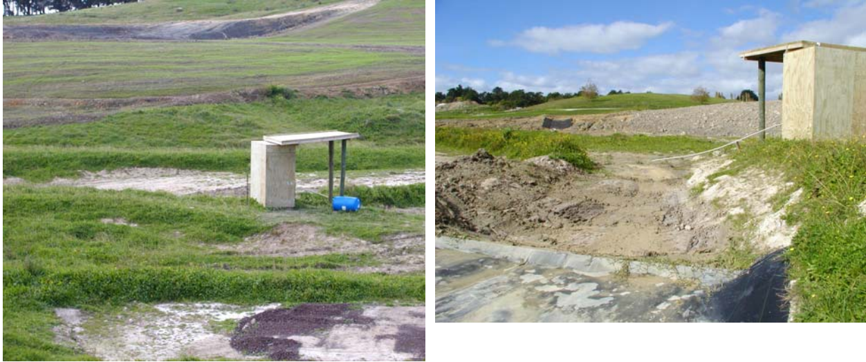
Figure 19. Auckland Regional Council rainfall-driven dosing system.
