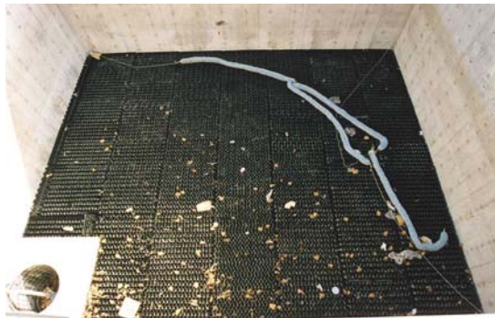
Lakewood Park and Ride, Caltrans, Los Angeles, CA, MCTT main settling chamber
