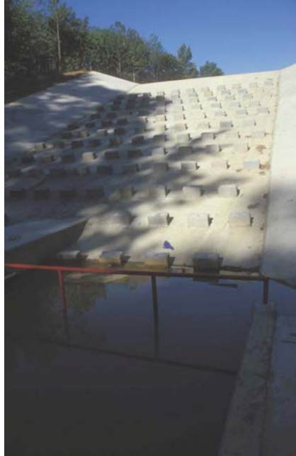
Large concrete emergency spillway with energy dissipater blocks
