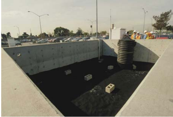
Lakewood Park and Ride, Caltrans, Los Angeles, CA, MCTT filtration/sorption chamber
