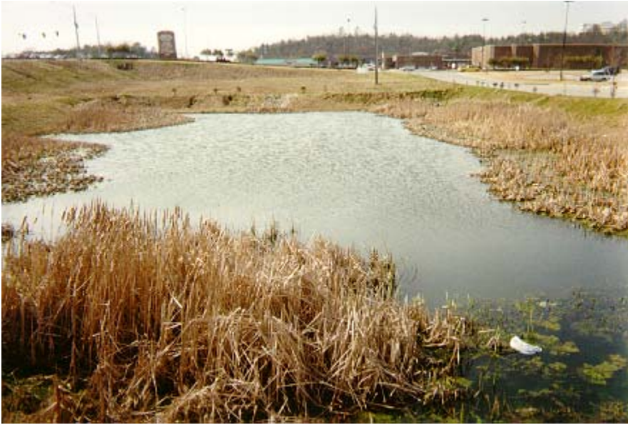
Figure 113. Facing west, inlets on right, obscured by cattails.
