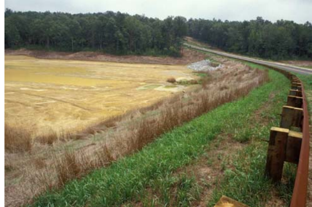
“Wet” pond built in area having Karst geology and sinkholes.
