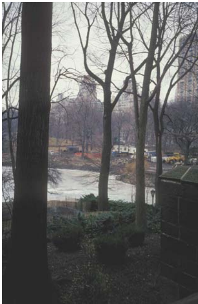
Central Park pond, NYC, being dredged and regraded
